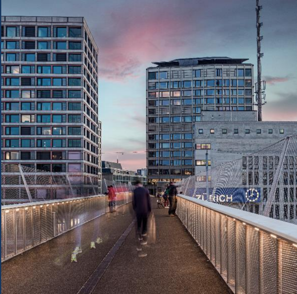
Developing both sides of the tracks reunites the city and its infrastructure
